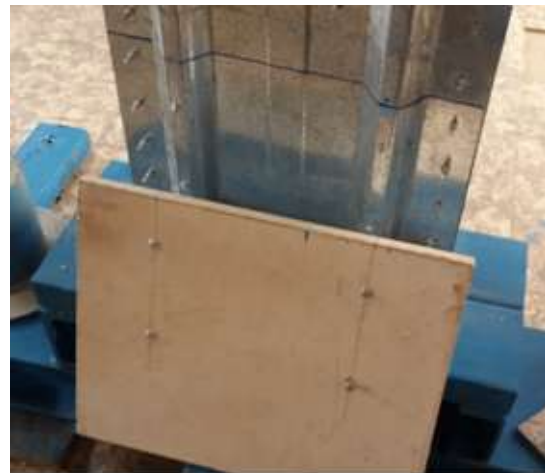
Figure (6) Shear Failure of connectors
