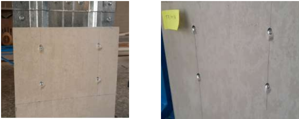
Figure (7) Failure of specimens by spalling of the dry board with the screws head still being attached
