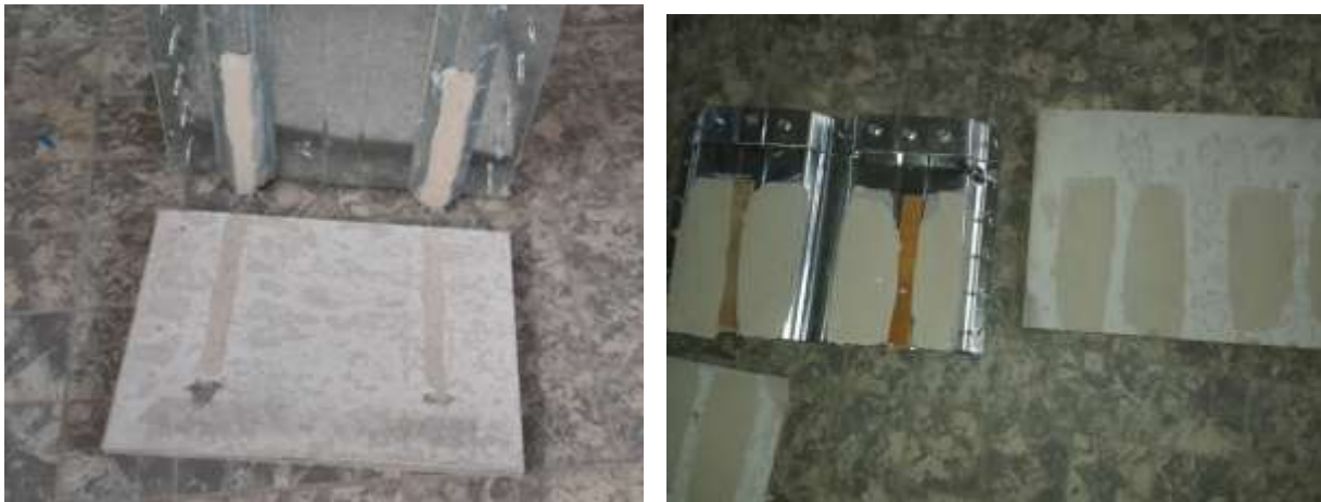
Figure (8) Failure of Specimens Connected by Epoxy by Separating The Dry Board From PSS
